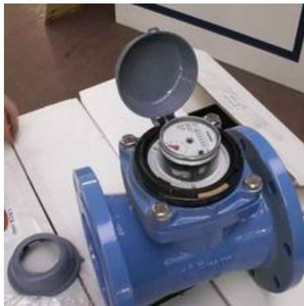
2) Remove the plastic ring
